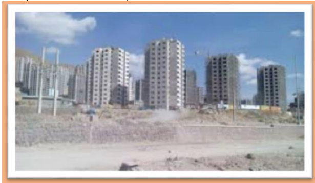
Figure 5: Pardis Mehr housing in suburbs area (URL 4).
