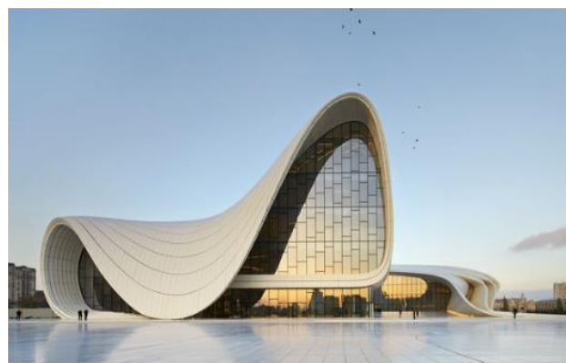
Fig.2: The representation of Heydar Aliyev Center Azaebarjan designed with advance composite material. Designing with advance composite materials opens up a wide range of design possibilities, it can also optimize the performance of a structure by the modification of the building blocks of the materials. The chemistry of the
